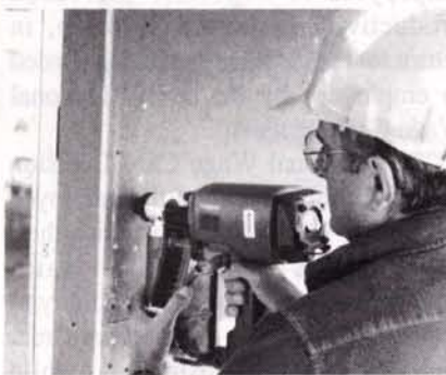
1/2" exterior gypsum sheathing fastened to nested (double thickness) steel stud. Below-flush application of interior gypsum board is made using special gypsum socket.
