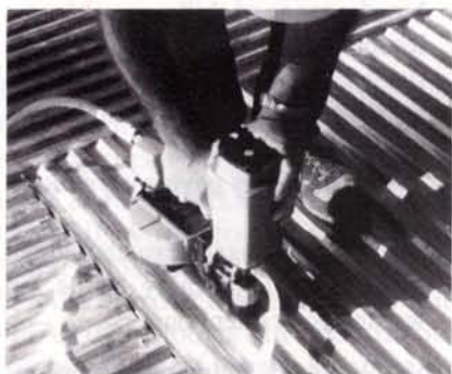
Fastening 26 gauge corrugated steel decking to 12, 14 and 16 gauge steel joists. Use standard socket.
