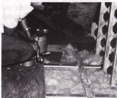
3/4" plywood sub-floor being fastened to 14 and 16 gauge steel joists. Use special toothed plywood socket for below-flush fastenings.
