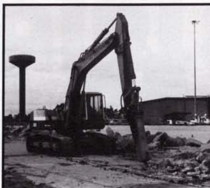
Baiaime demolishing a 14" of reinforced concrete.
